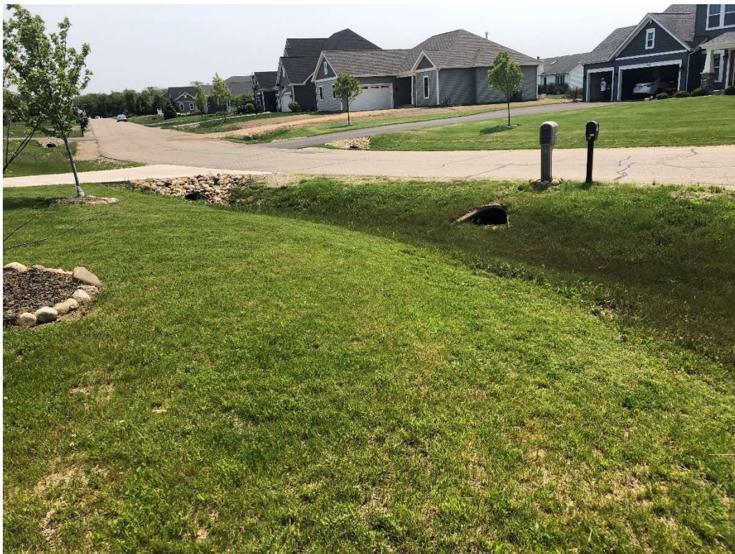
Westward Drive in front yard of Lot 2 showing historic water level.
