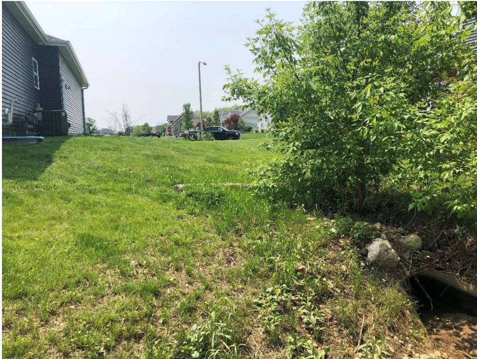
Photo looking toward Westward Drive from entrance to infiltration basin
