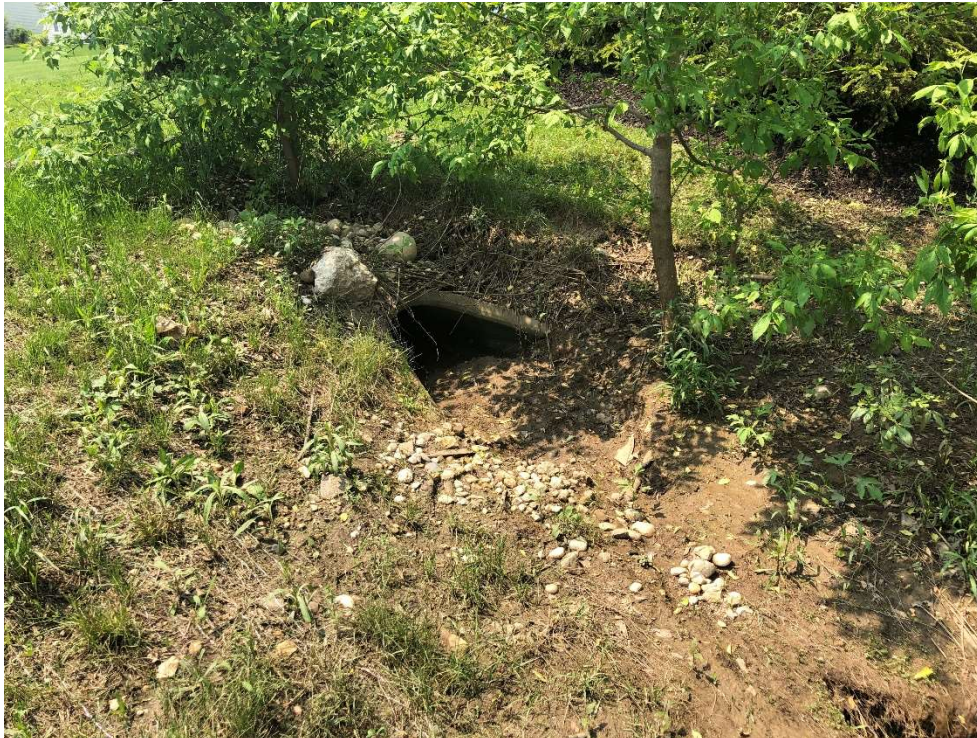
Entrance to infiltration basin showing vegetation and sediment fill materials
