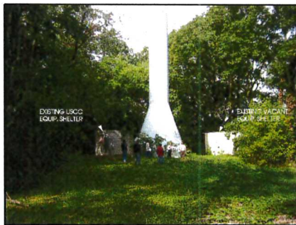
SITE OVERVIEW (LOOKING NORTHWEST)
