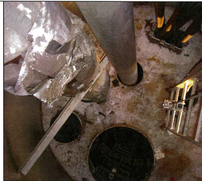
SECOND CONDENSATE FLOOR (LOOKING DOWN)
