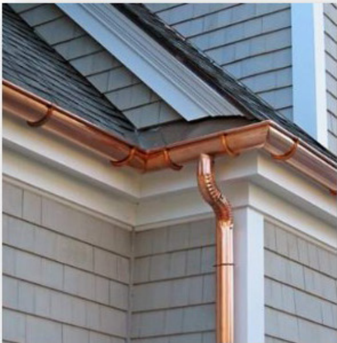
Half-round Gutters with Round Downspouts
