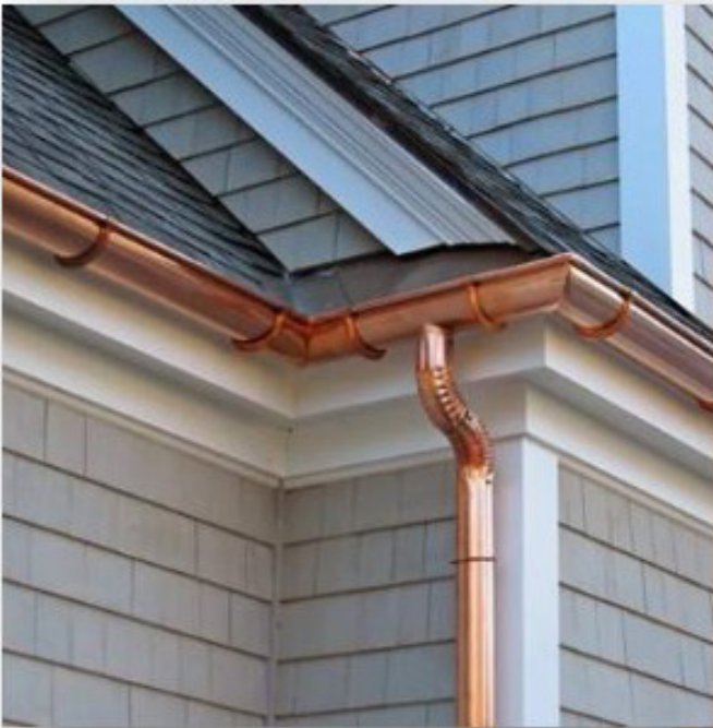
Half-round Gutters with Round Downspouts
