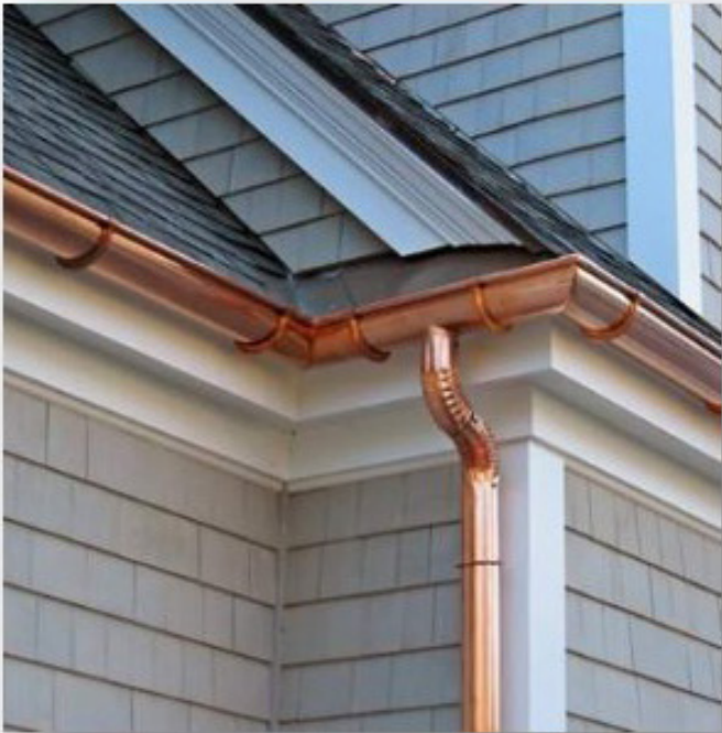
Half-round Gutters with Round Downspouts
