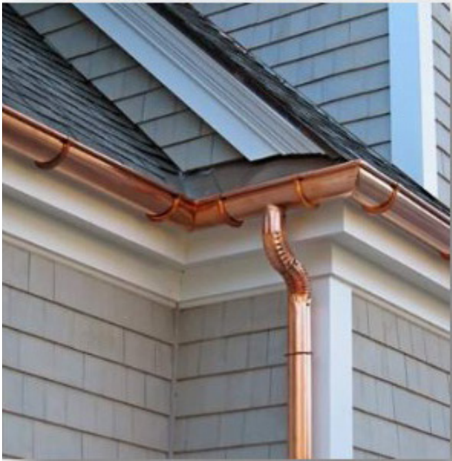
Half-round Gutters with Round Downspouts
