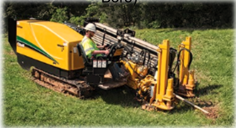
Buried Cable Placement (Directional Bore)
