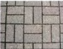
BASKETWEAVE PATTERN (2:1 RATIO) PROVIDES A FORMAL APPEARANCE SUITED FOR PEDESTRIAN AREAS
