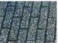
RUNNING BOND PATTERN PROVIDES A FORMAL APPEARANCE BEST SUITED FOR PEDESTRIAN AREAS
