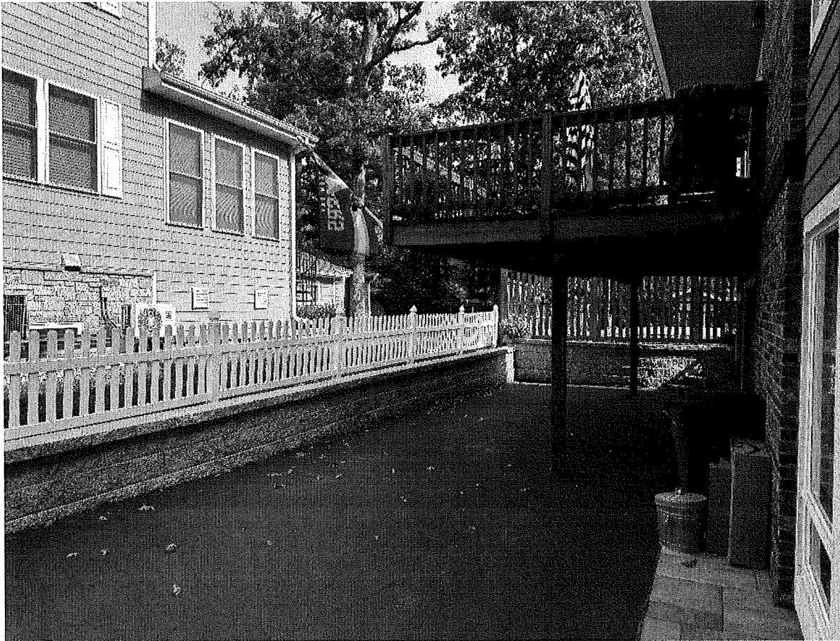
Exhibit 4. Picture of the driveway looking East from driveway at retaining wall.
