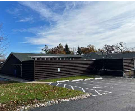
Existing dining facility and kitchen
