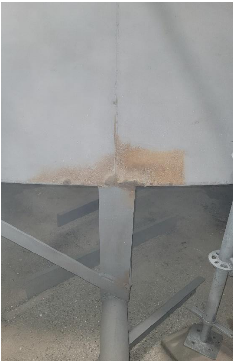
Porosity in overlapping seams.
