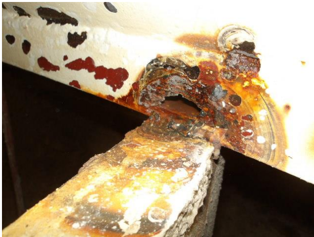
Advanced corrosion prior and post blasting.
