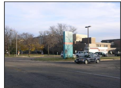
Aurora Lakeland Medical Center in the City of Elkhorn
