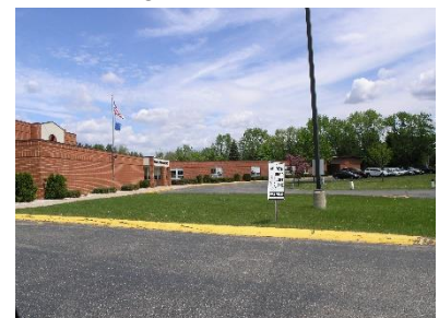
Tibbets Elementary School in the Town of Sugar Creek
