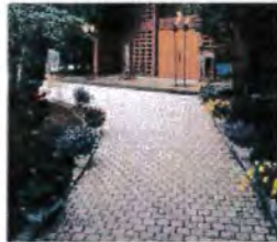
TUMBLED LIMESTONE PAVERS INCORPORATED INTO A PEDESTRIAN WALKWAY
