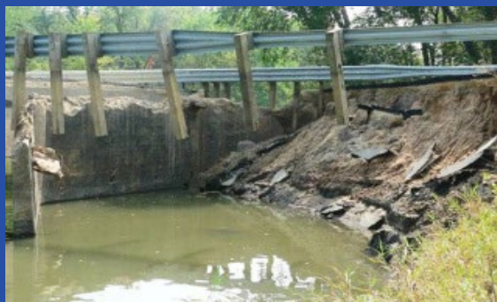
C. Roads & Bridges
