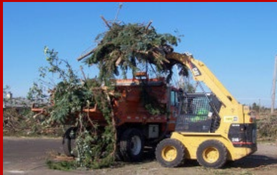
A. Debris Clearance
