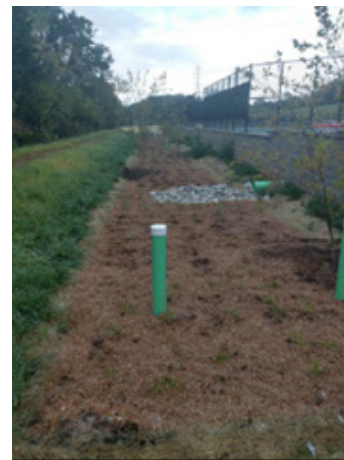
Figure 9. An image of a finished trench. 8
